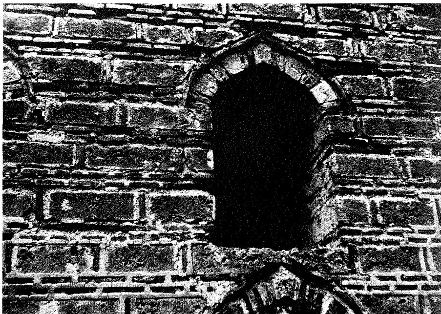
18 — Banitsa, Village Mosque, detail of masonry.
